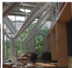
Lillis School of Business, University of Oregon, LEED Gold
