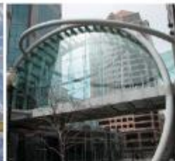
Pedestrian Bridge, Salt Lake City
