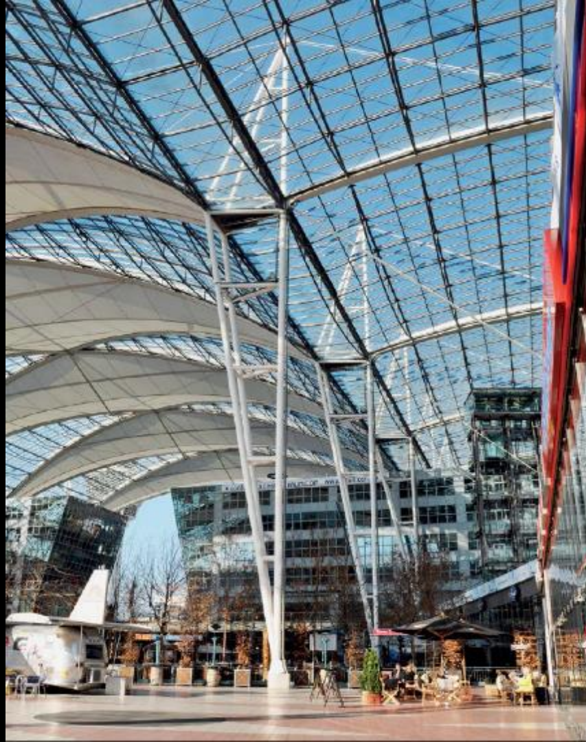
The Munich Airport Terminal in Munich, Germany, designed by Helmut Jahn and completed in 1991, showcases high-level detailing in Architecturally Exposed Structural Steel.
