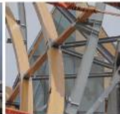
Art Gallery of Ontario, Frank Gehry (for steel and wood)
