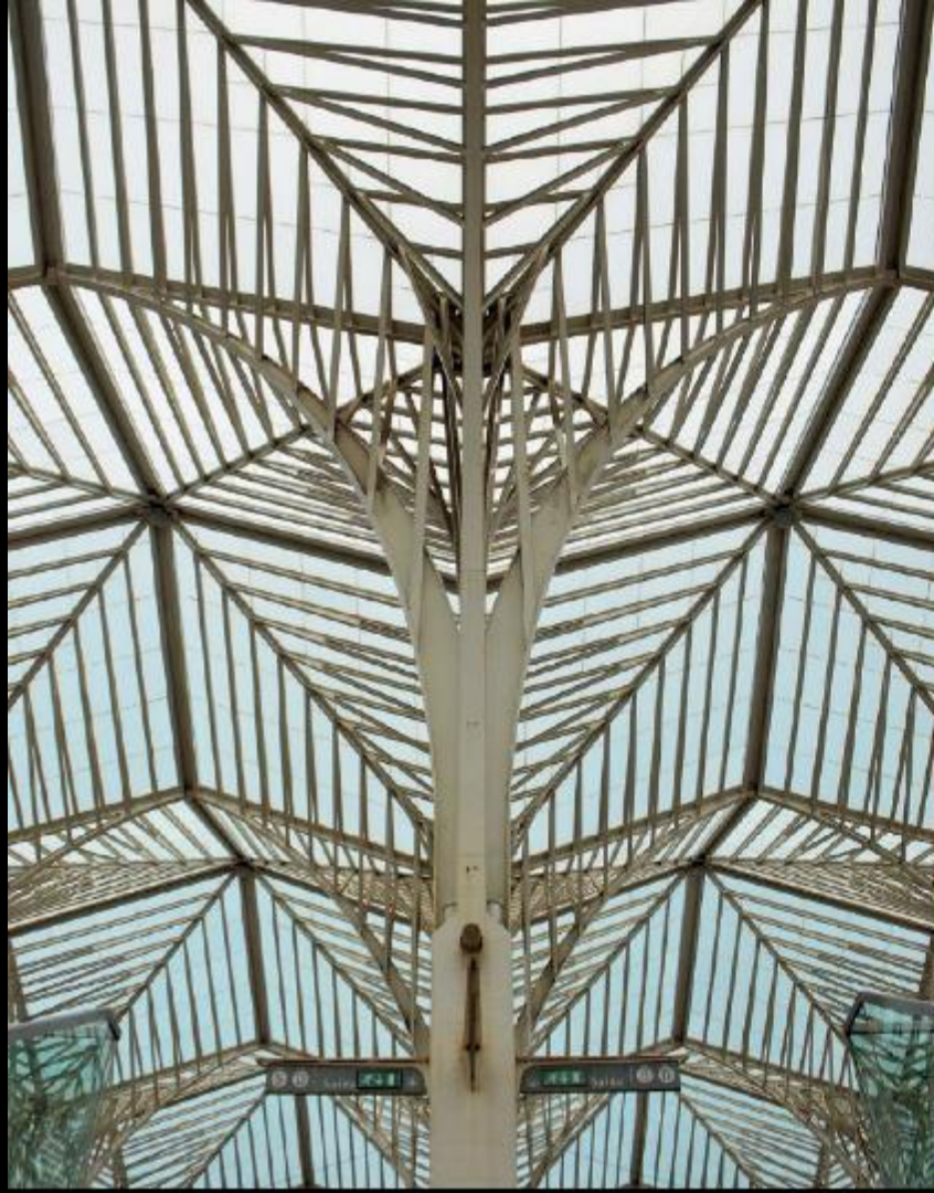
Member Section in Union, Portugal, designed by Santiago Calatrava, constructed for Expo '98, stands as a project that left a profound impression on AESS. The complexity of the fabrication was unprecedented for any steel structure at the time. A project that has been included in chapters to using a variety of types of steel and structural and fabrication details.
